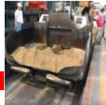
Mixed Soil Paving By Finisher
